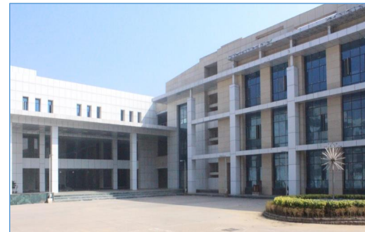
NCRB new building at Mahipalpur, Delhi
